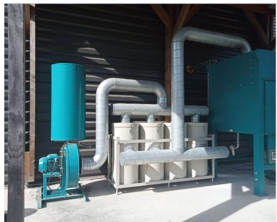
FIGURE 39 : AIR EXTRAIT DE LA MACHINE DE DECOUPE LCD – UNITE TRAITEMENT DE L'AIR
